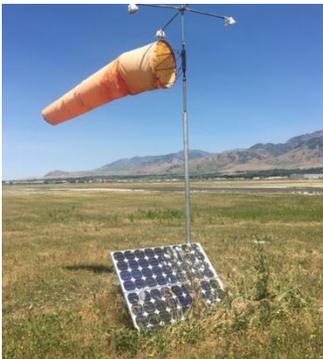
Wind-cones installed (solar) are very dim, and difficult to see. Determine if all (solar) wind cones meet the photometric requirements of 150/5345-27. If not, develop a plan to replace. In addition, supplemental wind cones were faded and require replacement.
